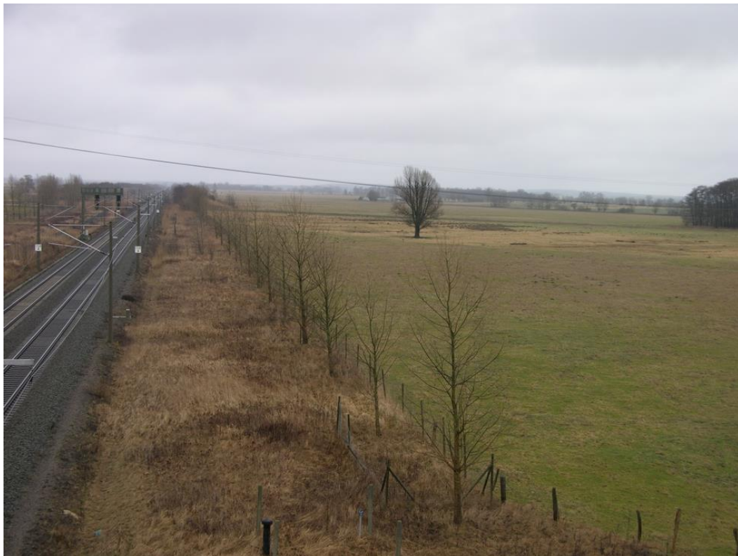
Figure 7: Planted shelterbelts in the Havelländisches Luch Great Bustard habitat, in Germany for „covering” the railway electric cables. Photo: Eike Julius.
