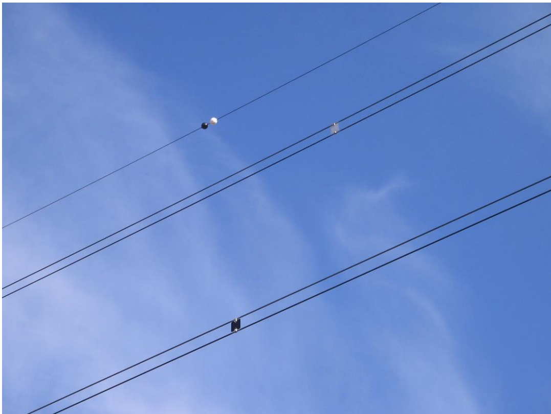
Figure 6: bird protection balls and bird protection plates (Photo: R. Raab) on high voltage power line in Austria.
