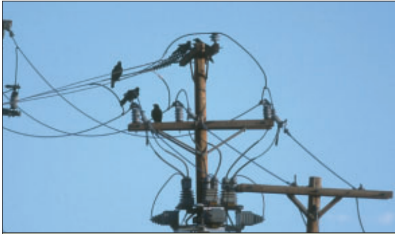
FIGURE 4.15: Numerous birds perched on a pole can increase electrocution risk. Pictured: common ravens during breeding season.
