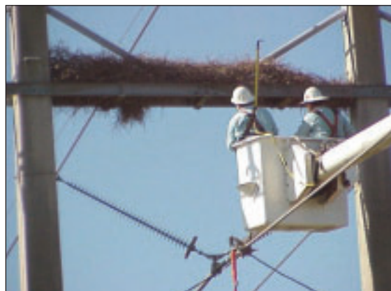
FIGURE 6.8: Monk parakeet nests on transmission tower.
