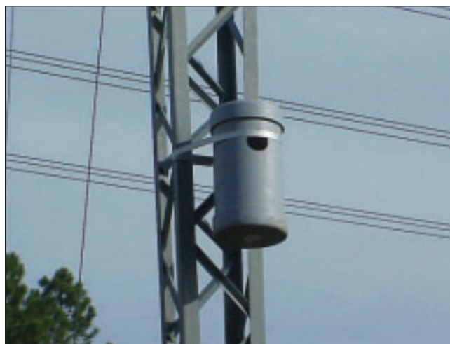
FIGURE 6.20 Kestrel nesting tube (46-cm [18-in] length) installed on transmission tower in Georgia.
