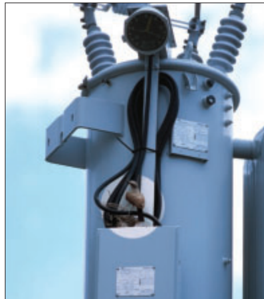
FIGURE 6.7: Western kingbird nest (see highlighted area) on transformer.
