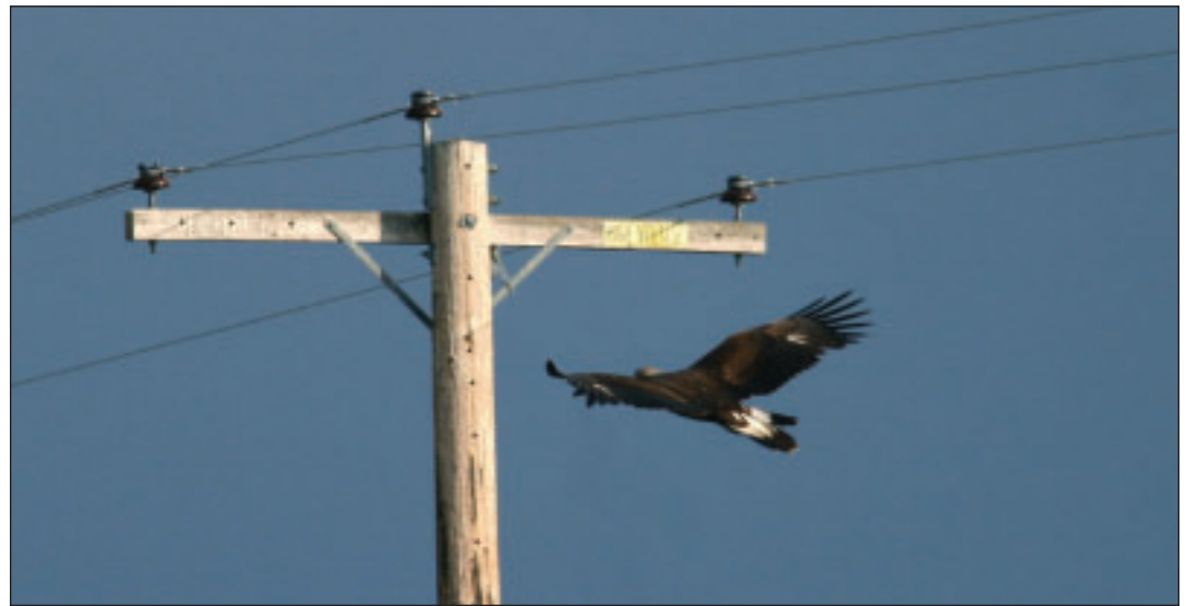
FIGURE 4.14: Juvenile golden eagle about to land on a distribution pole that is not avian-safe.
