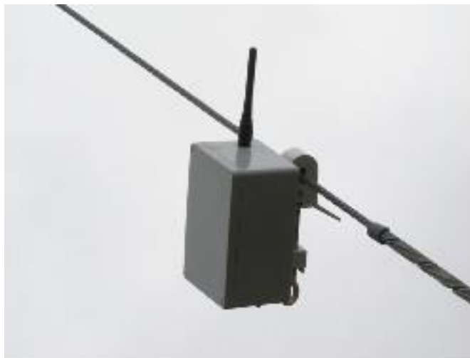
Figure 3.1 Bird Strike Indicator (BSI) attached to a power line. BSIs are relatively small devices that can be attached to a single wire of a power line and automatically register bird collisions based on the vibration of the wire.
