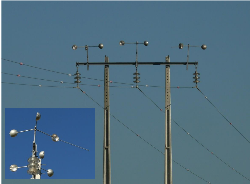
Figure 2.5 Perching dissuasion devices to prevent White Storks from nesting on utility poles in Portugal (Photo: H. Prinsen).
