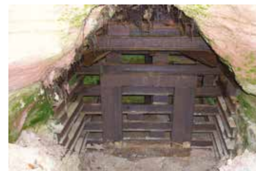
Large-section grille, Lambertsberg, Germany.
