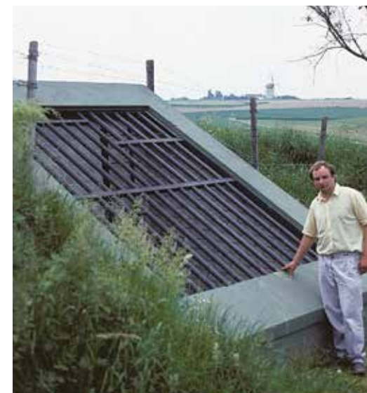
Large grilled mine, S. Limburg, The Netherlands.
