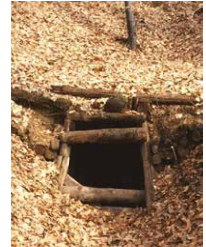
Király-bányák mine entrance before reconstruction.
