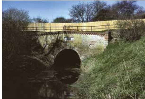
Greywell canal tunnel grille.
