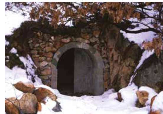
Király-bányák mine entrance after reconstruction and improvement.
