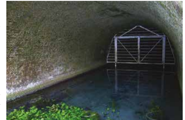
Entrance to Greywell canal tunnel.
