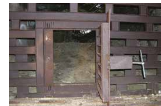
High-security entrance door, Gauberg, Germany.
