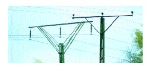
Only the power pole with suspended insulators is safe. Mitigation measures to protect birds from electrocution will pay off only if carried out consistantly and on a large scale.
