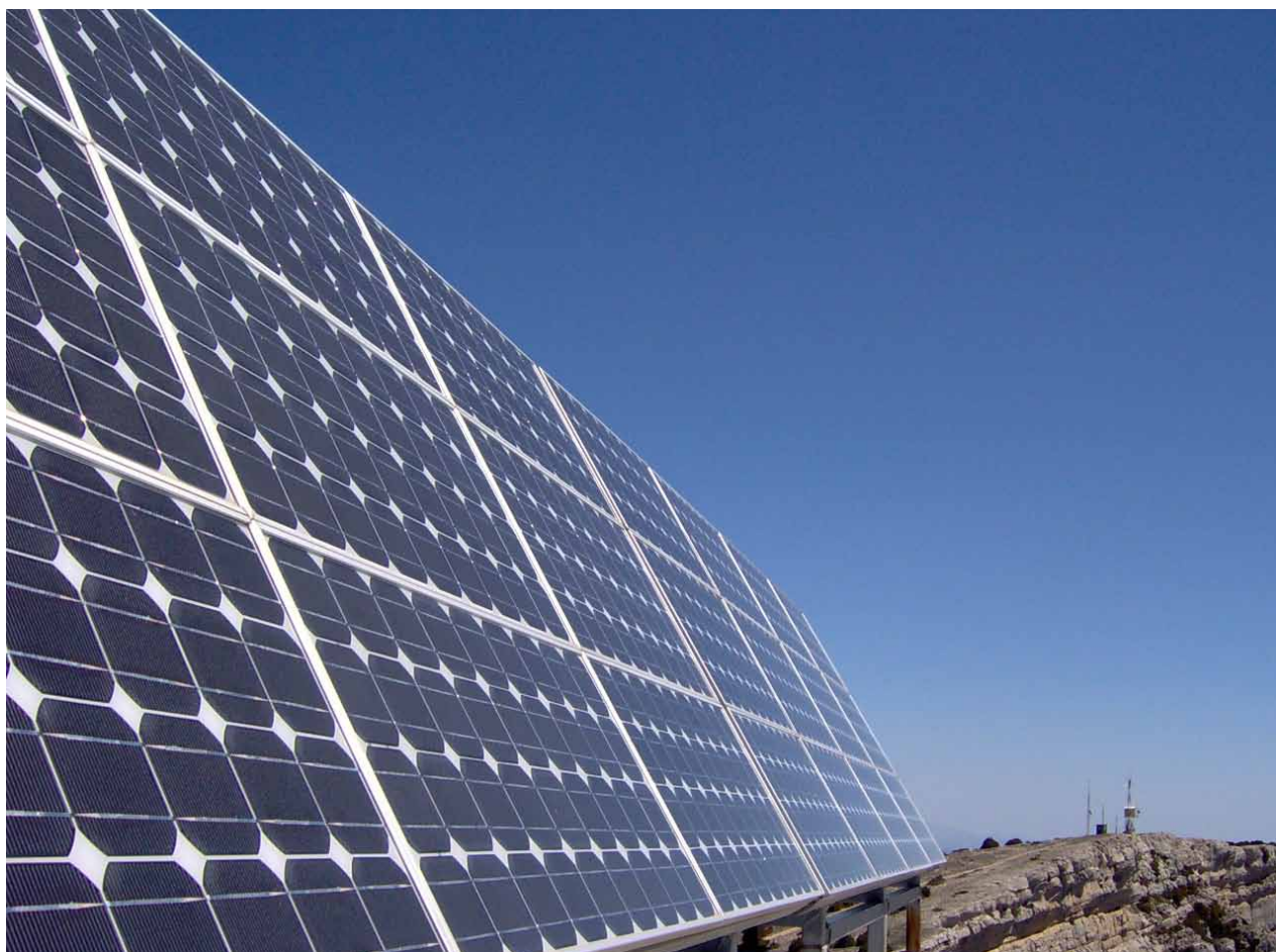
Installation solaire © Fernando Tomás/Flickr
