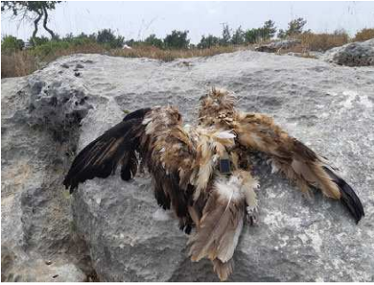
Bird mortality caused by the power lines in southern Turkey.
