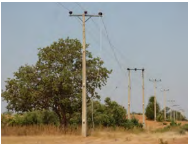
Survey of power lines in Nigeria.
