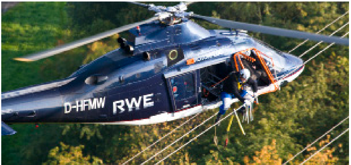
Installation of bird flight diverters by helicopter on a high voltage power line in Germany © RWE Rhein-Ruhr Netzservice
