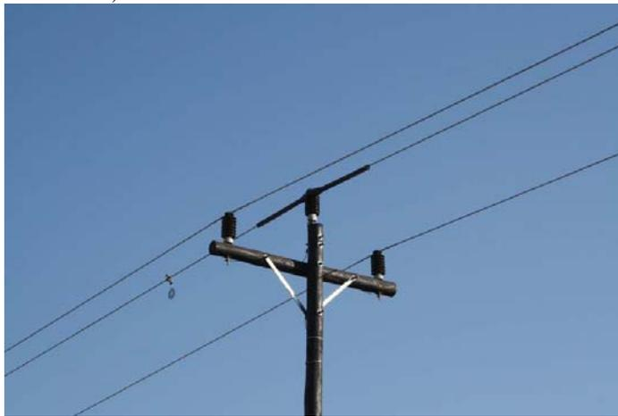
Figure 13. A 'Raptor Protector' used to insulate the centre conductor of a 22 kV pole structure making the distances between non-insulated conductors large enough for safe perching (Photo: EWT-WEP).
