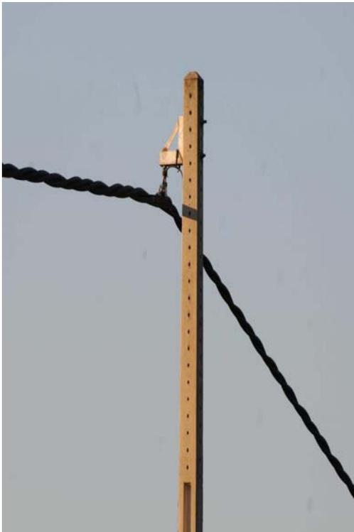
*Figure 9. Completely insulated medium tension cable in Spain hanging from concrete pole without need of insulators (source: Haas, 2011).*
