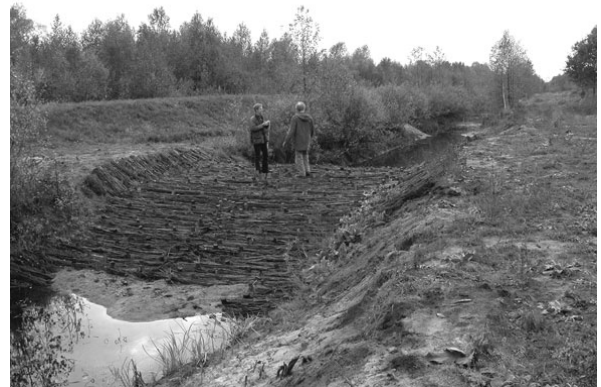
One of the dams at Zvanets
