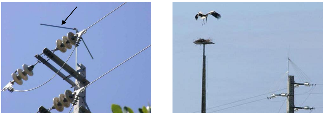
Figure 5. Distribution pole with symmetric chevron (arrow) on top as bird exclusion device (Photo: EDP-Distribution, Portugal) and dedicated nesting pole for White Stork next to distribution pole with bird exclusion device (Photo: Carlos Tiago).
