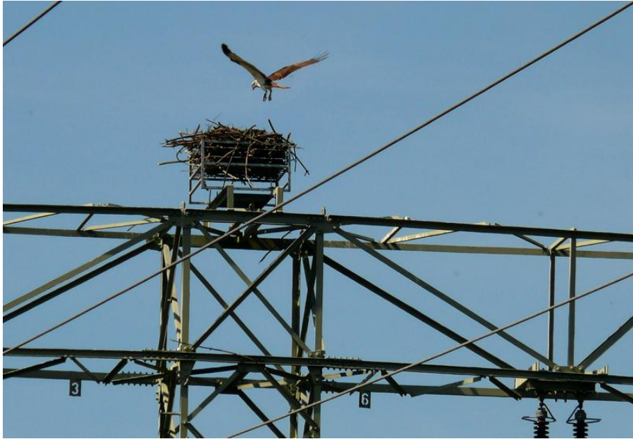
Figure 13. Nesting Osprey on artificial platform in medium voltage transmission line, Muritz National Park, Germany (Photo; Bureau Waardenburg).
