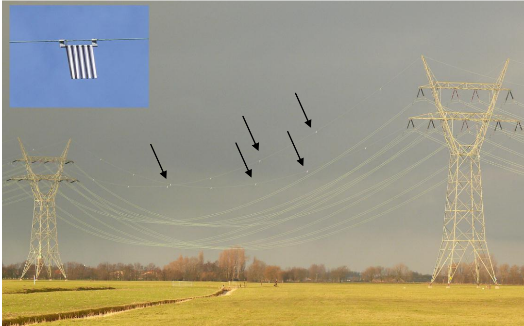
Figure 12. High-tension (150 kV) power line in the Netherlands with bird flappers (inset) (see arrows) placed at regular intervals in both ground wires as bird flight diverters, see also Box 1 (Photo: Bureau Waardenburg).
