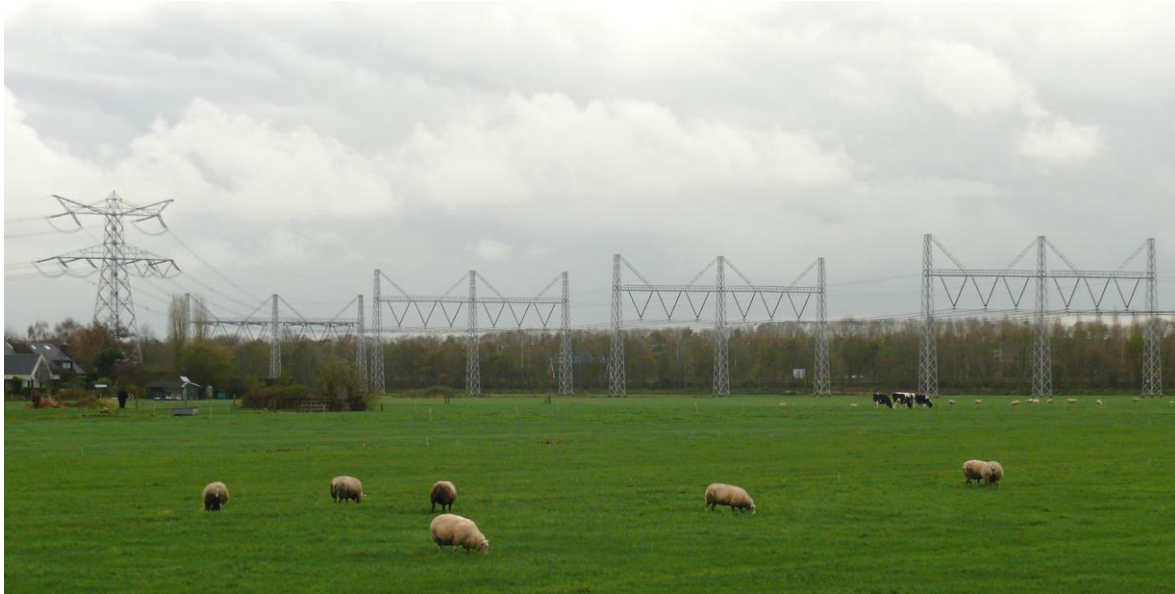
Figure 7. A 380 kV line, with lowered conductor wires hanging from portals in one horizontal plane to minimise collision risk for Great Cormorant ( Phalacrocorax carbo ), Eurasian Spoonbill ( Platalea leucorodia ) and Purple Heron ( Ardea purpurea ) daily passing this stretch of line while commuting between the breeding colony and foraging areas, Muiden, the Netherlands (Photo: Bureau Waardenburg).
