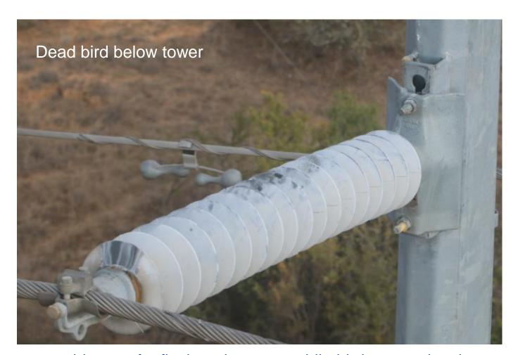
Apparent evidence of a flash to the tower while bird was on insulator
