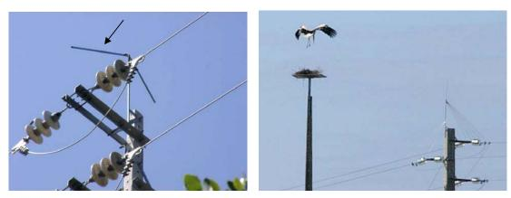
Figure 11. Distribution pole with symmetric chevron (arrow) on top as bird exclusion device (Photo: EDP-Distribution, Portugal; and distribution pole with bird exclusion spikes with dedicated nesting pole for White Stork next to it (Photo: Carlos Tiago).
