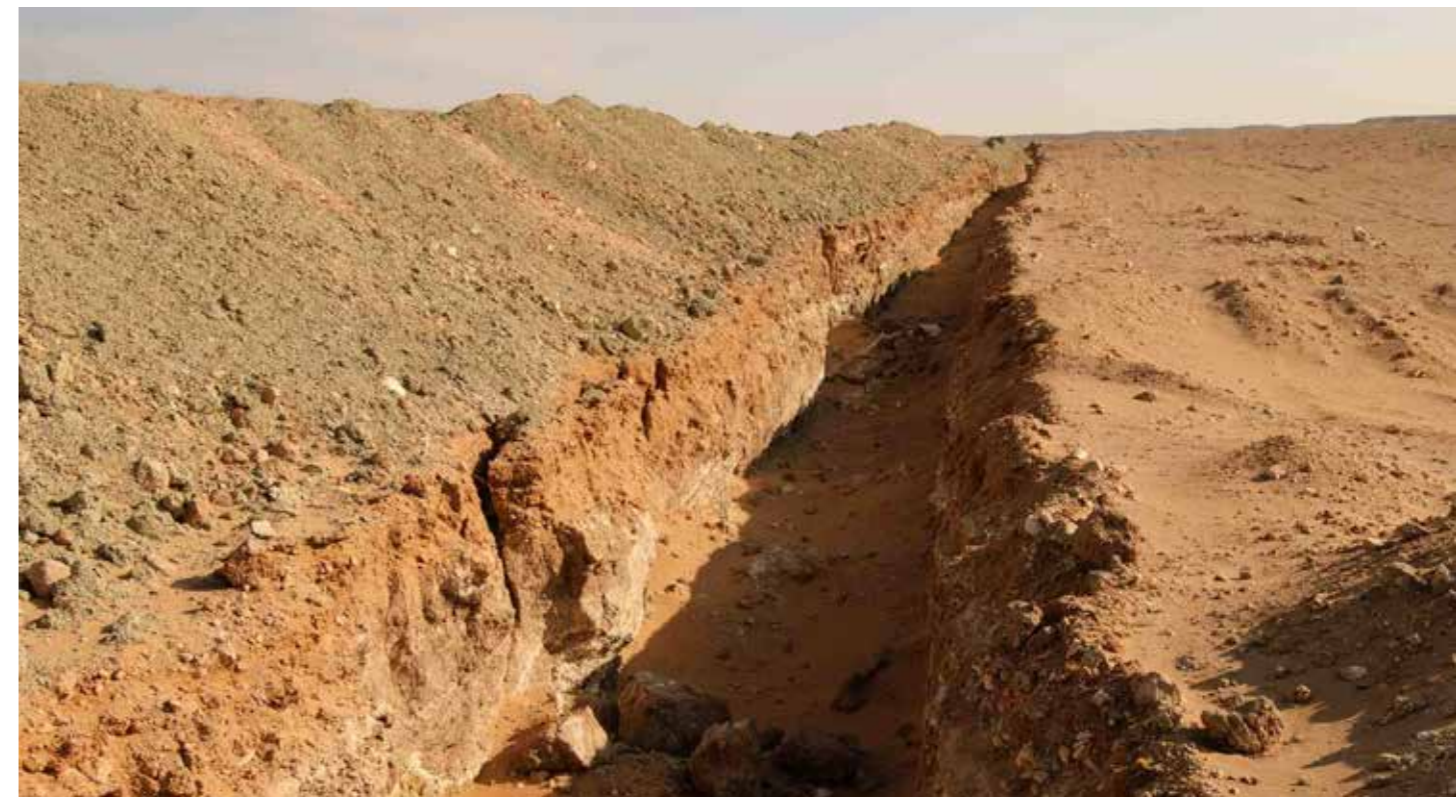
Ditches created during the construction of pipelines or as a measure to prevent vehicles from leaving established roads represent another hazard and potential barrier to wildlife movement. ©WCS/K. Murphy
