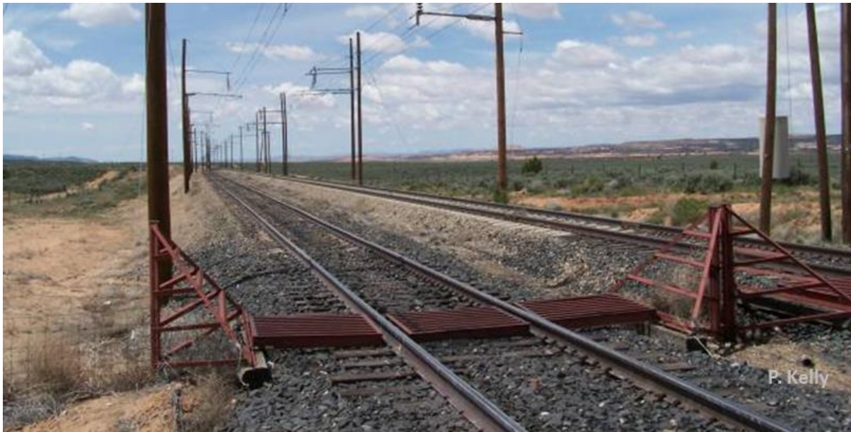
Figure 31. A railroad cattle guard prevents animals from walking on the tracks which reduces train strikes.
