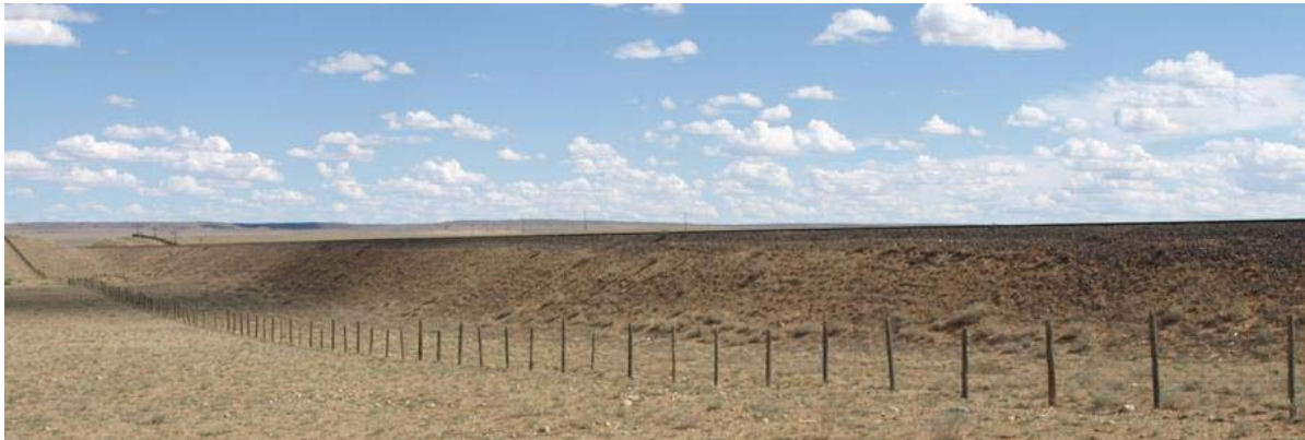
Figure 5. This embankment is about 3 meters high and might be enough to prevent movements of gazelles and other open plains animals to the other side.
