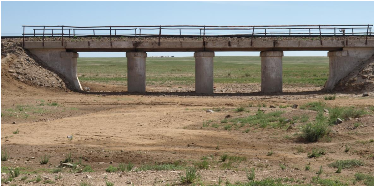
Figure 23. A typical bridge design over an intermittent drainage along the Trans Mongolian Railroad.
