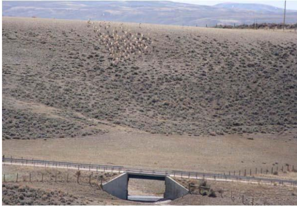
Picture 3 . Road underpass in USA
