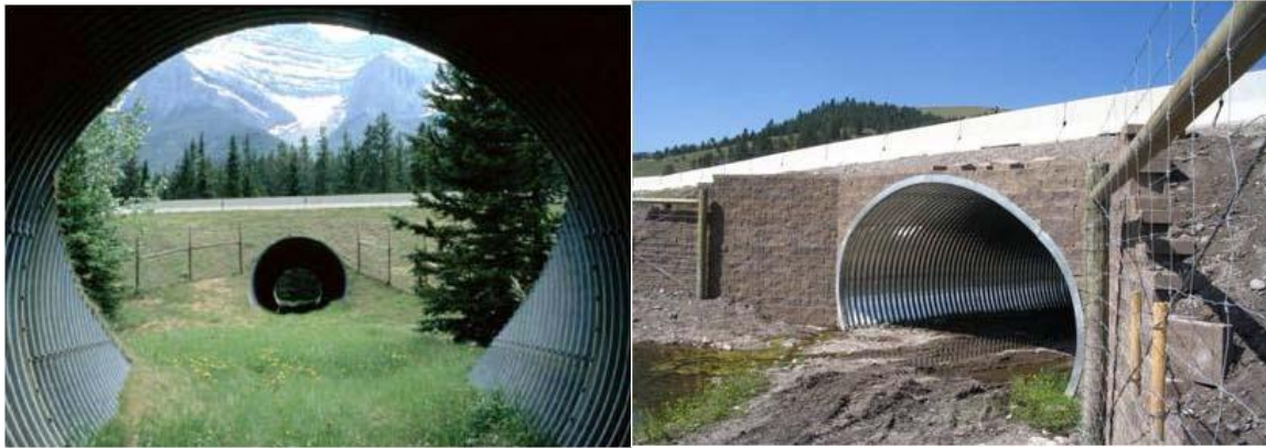
Pic. 7. Suggested wildlife friendly underpasses underneath road.
