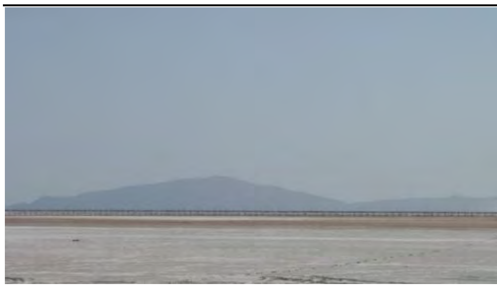
Figure 9.74 Previous Semi-Mechanised Salt Projects (pumped saline pipeline to evaporation ponds)
