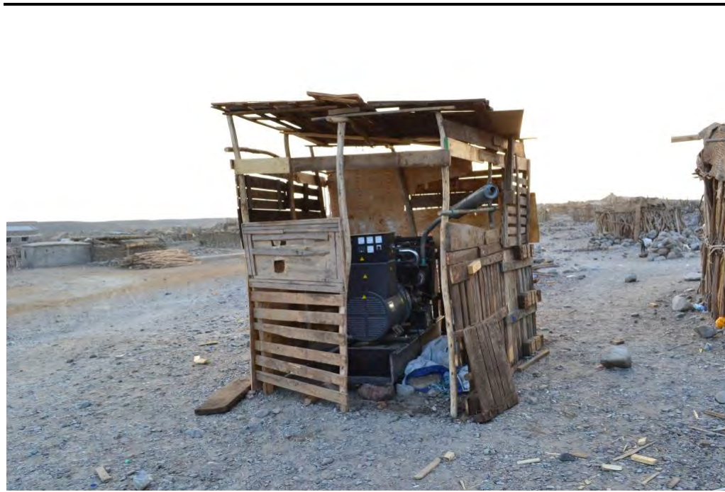
Figure 9.17 Diesel Generator in Hamad Ela
